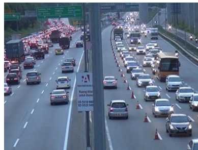
Fig.3: Traffic cones lane splitter at KESAS Expressway
