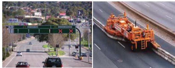
(a) Lane control lights (b) Barrier Transfer Machine
