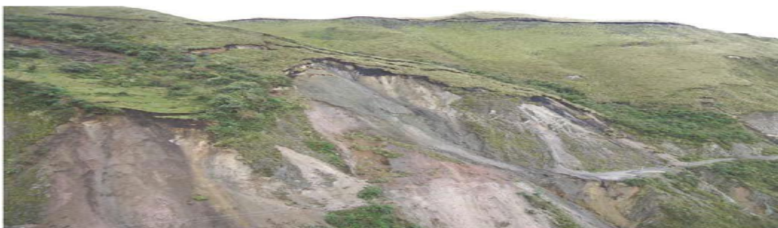
Figure 1. The landslide that affected the headrace tunnel [Source: Micheli et al., 2013]
