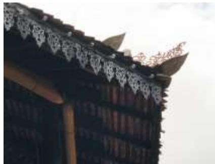
Figure 3 Roof ornamentation (source author)
