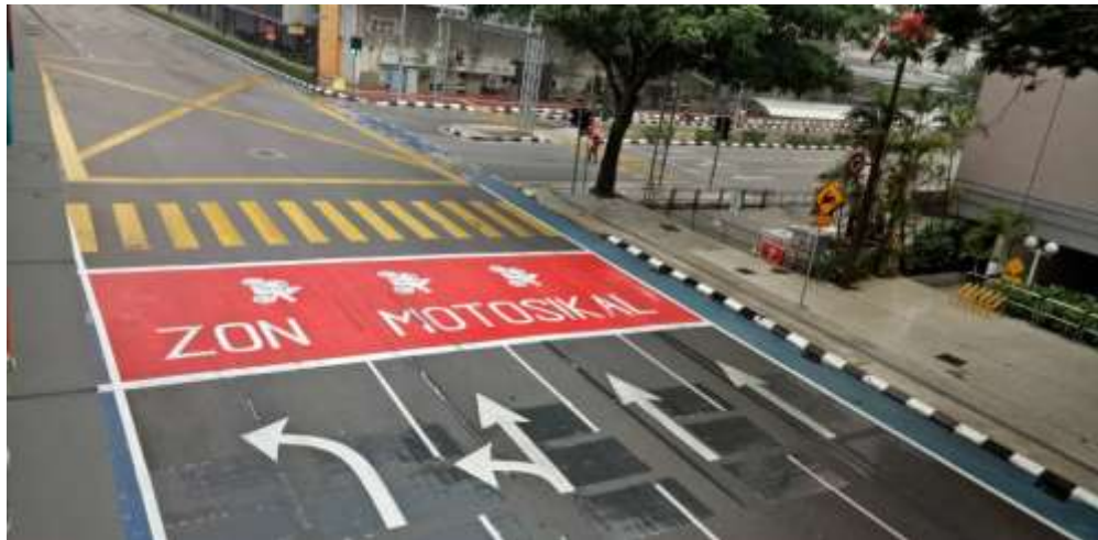
Figure 1: The example of an ASL for motorcycle at one of the signalised intersection in Kuala Lumpur
